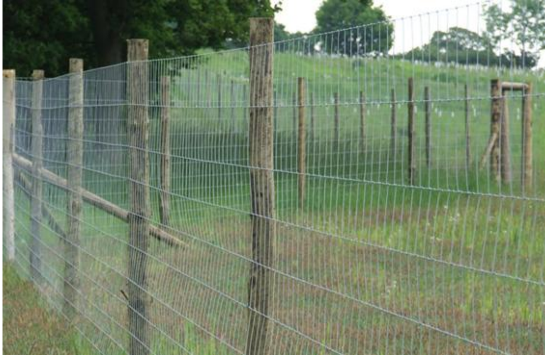
Plate 3-9: Typical stock proof security fence
