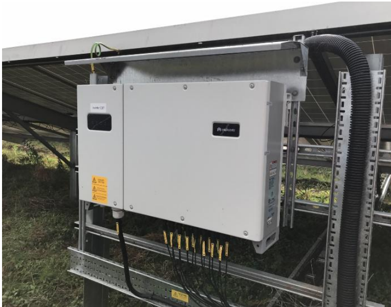
Plate 3-4: Typical string inverter (image reproduced courtesy of Huawei)
